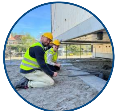
Assemblage on site door lokaal assemblageteam
